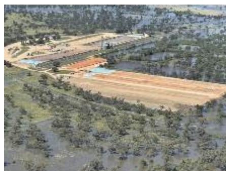
Bunker Grain silo north of Walgett
